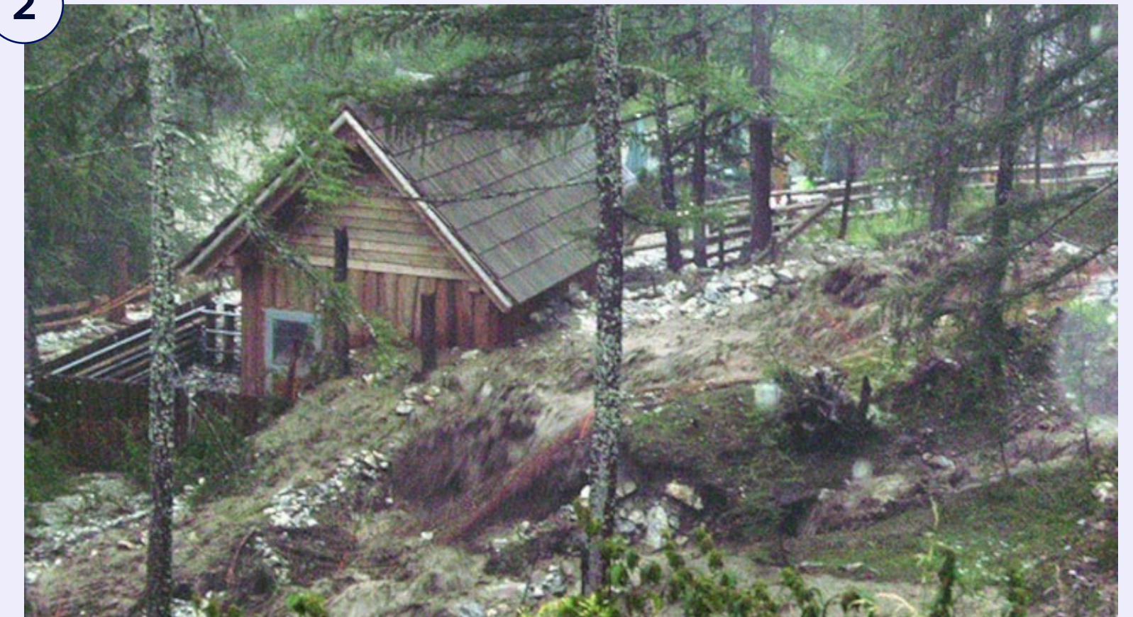
Landslide in the Riedingtal, 2015
